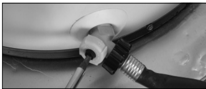
Figure 41 - Draining the water heater.
