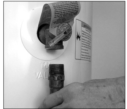
Figure 21 - Removing the T&P Relief Valve discharge pipe.
